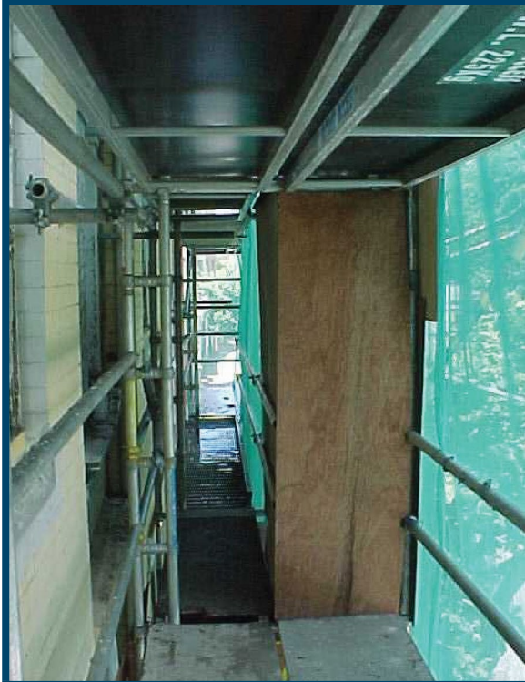
FIGURE 2 Enclosure on internal side of the scaffold
